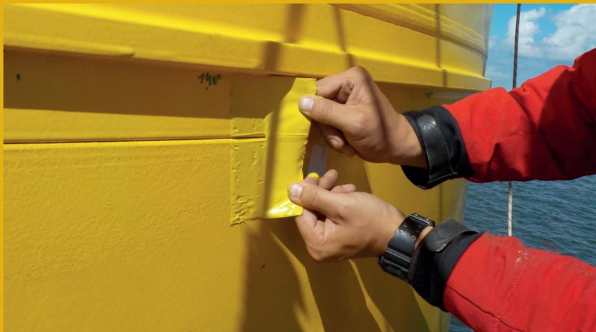
all it takes is a wire brush, a piece of the Coating Repair Patch that is already pre coated, add to the substrate and the job is done. It's as simple as applying a structural band aid if you can call it that.
