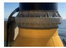
An offshore crane flange protected with the Oxifree coating solution
